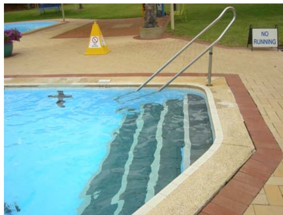
A graded step entrance and pool chair lift (not shown) makes access to the Boyup Brook Swimming Pool easy for all
